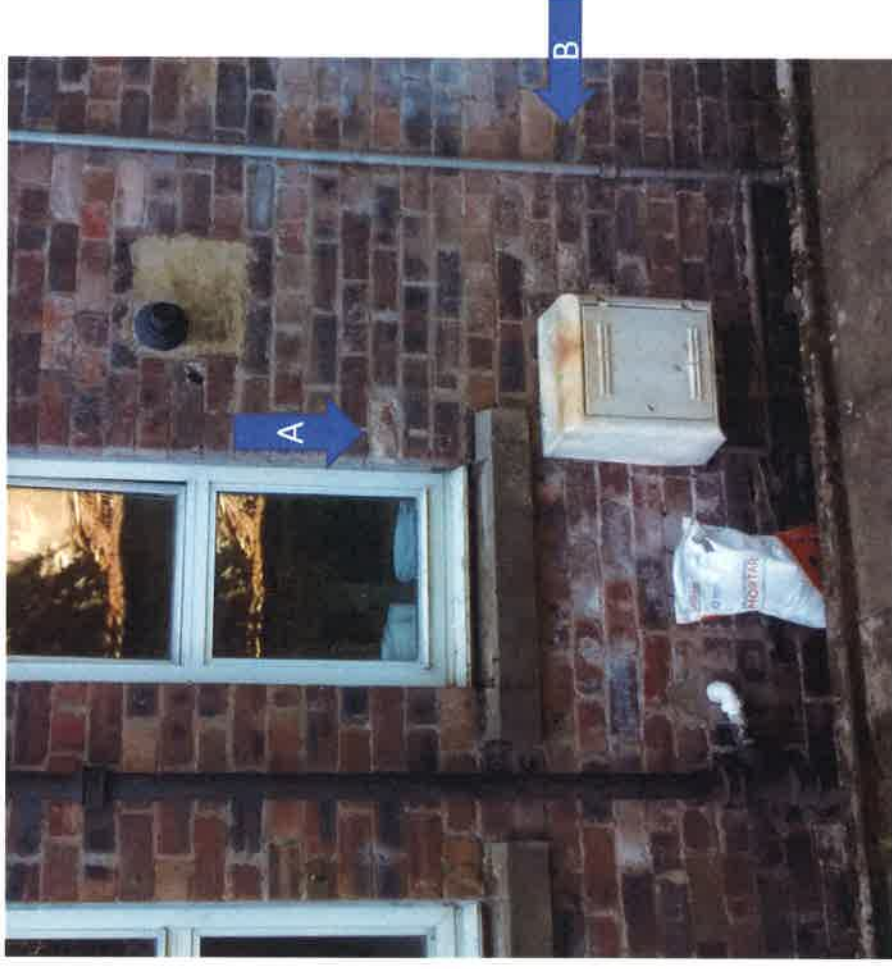
As at 31/04/17 – some repointing carried out, but the standard and extent of the work is poor (see also 3b).
