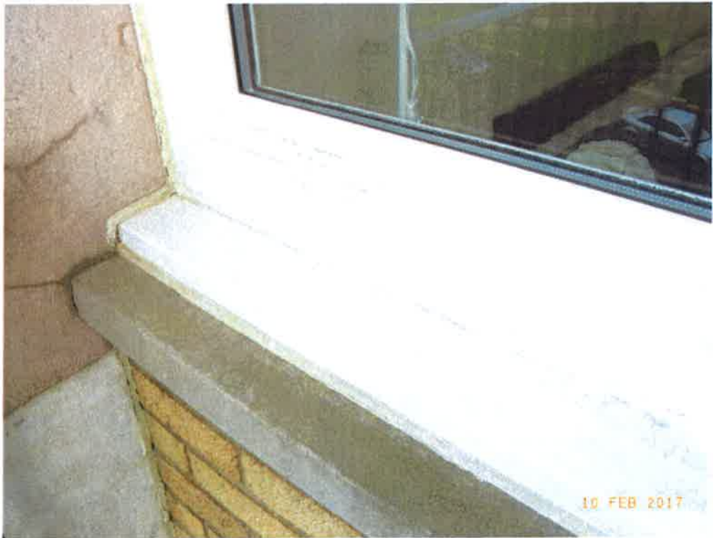
Lounge window – exterior
