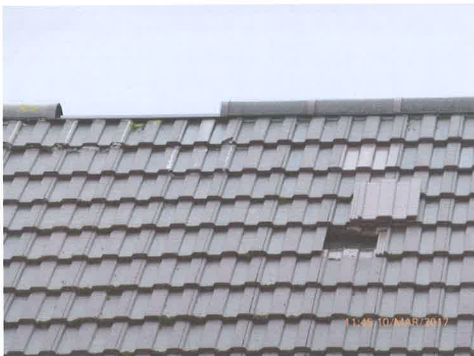
Missing/dangerous roof tiles
