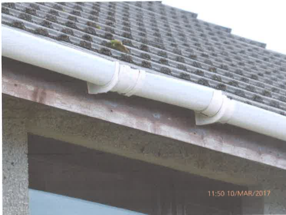
Defective guttering
