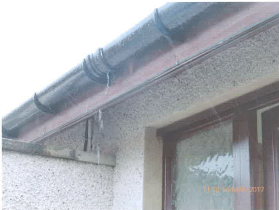
Leaking gutter
