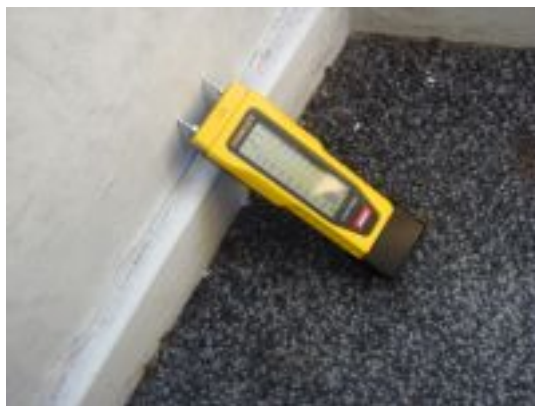
Meter reading at front wall of bedroom(0.6)
