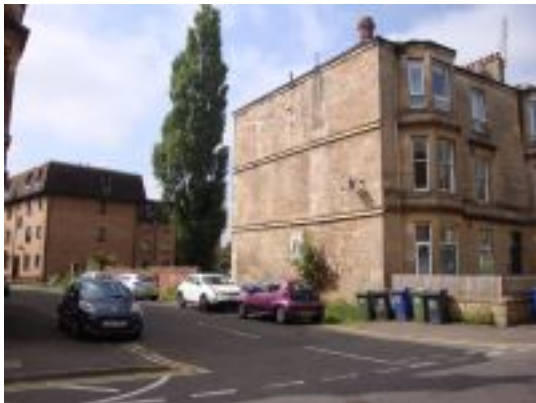
Exposed gable wall
