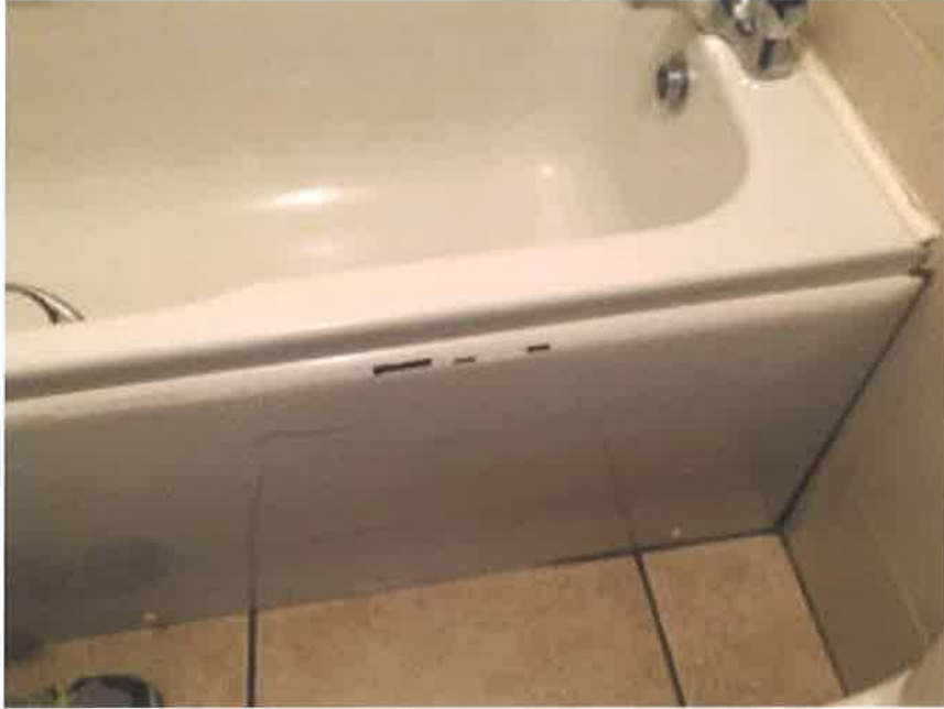
7. Damaged bath panel in the main bathroom.
