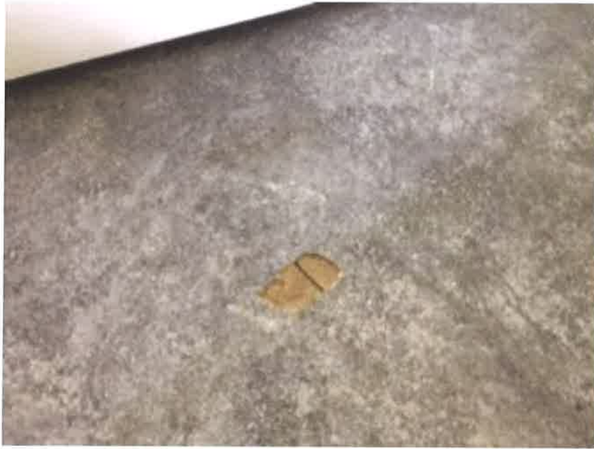
3. The defective vinyl flooring in the kitchen.
