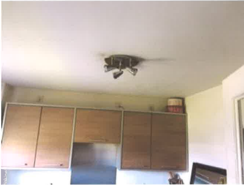
5. No heat detector in the kitchen.
