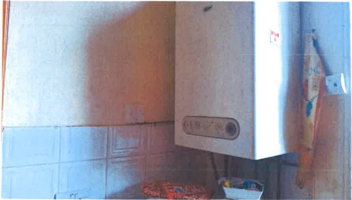
Boiler in kitchen – replacement power supply, and position of carbon monoxide monitor.
