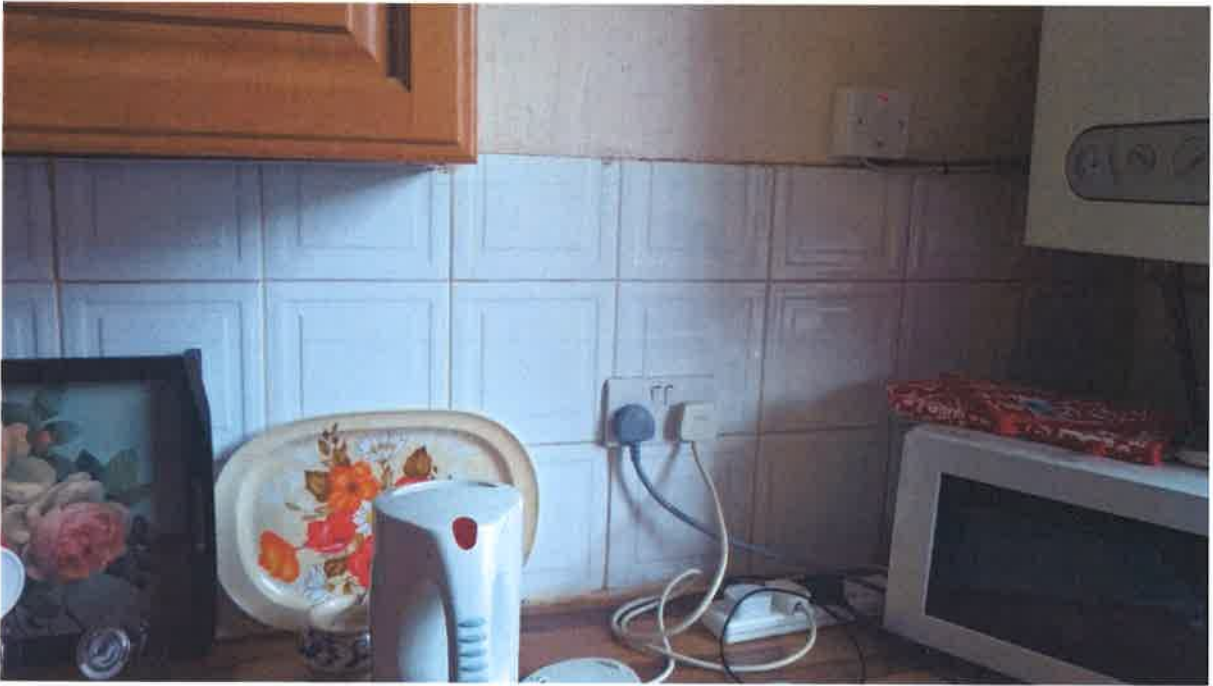
Replacement electrical socket in kitchen
