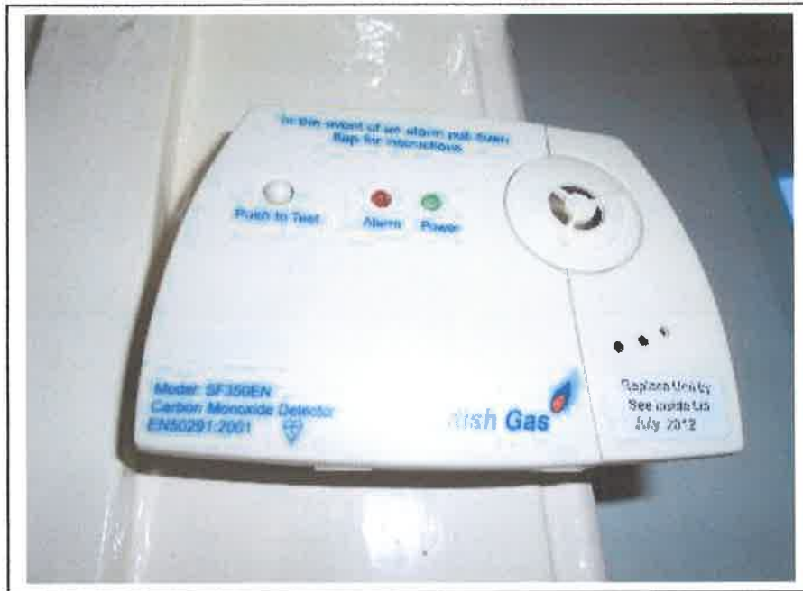
Carbon Monoxide monitor located in hallway – not operational.
