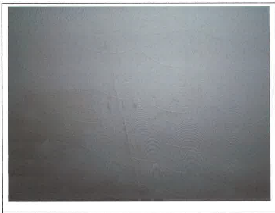
Damp staining in bedroom partially redecorated
