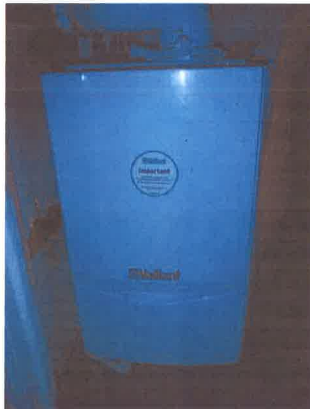
Photographs 3 and 4: Rear bedroom - Vaillant gas boiler
