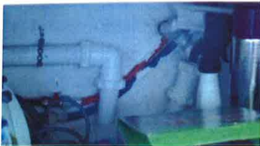
Photo 5 – Repaired waste water pipe
