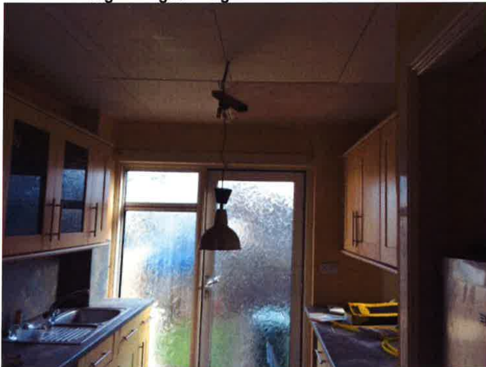
Kitchen ceiling and light fitting
