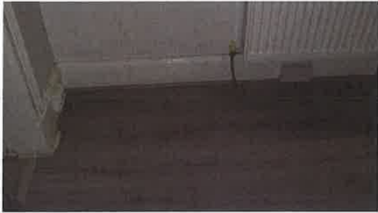
Photo 8 – New flooring in Hallway
