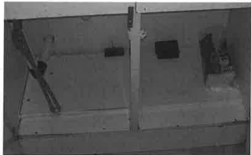
Photo 3 – Kitchen sink cupboard
