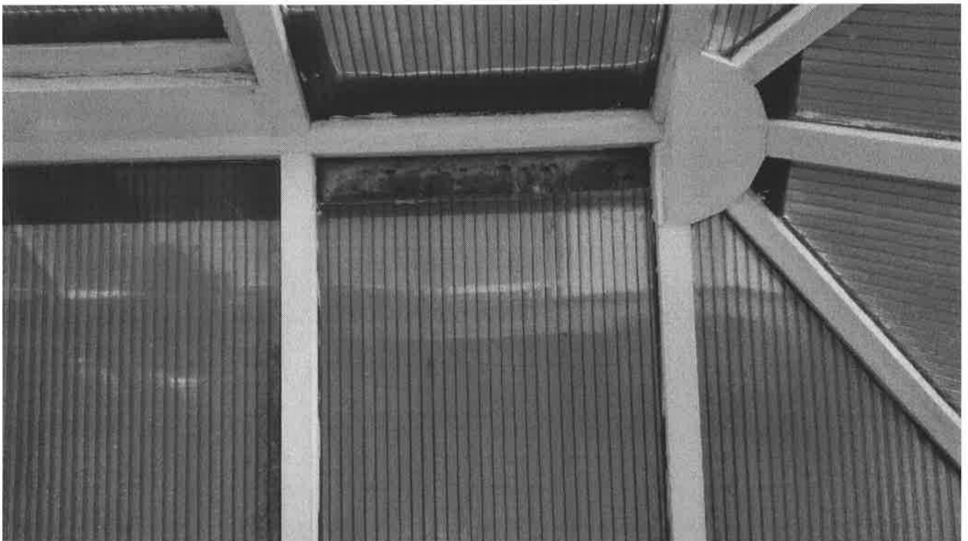
1e) Right slipped glazing panel exposing the flashing
