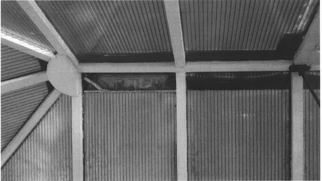
1e) Right slipped glazing panel exposing the flashing
