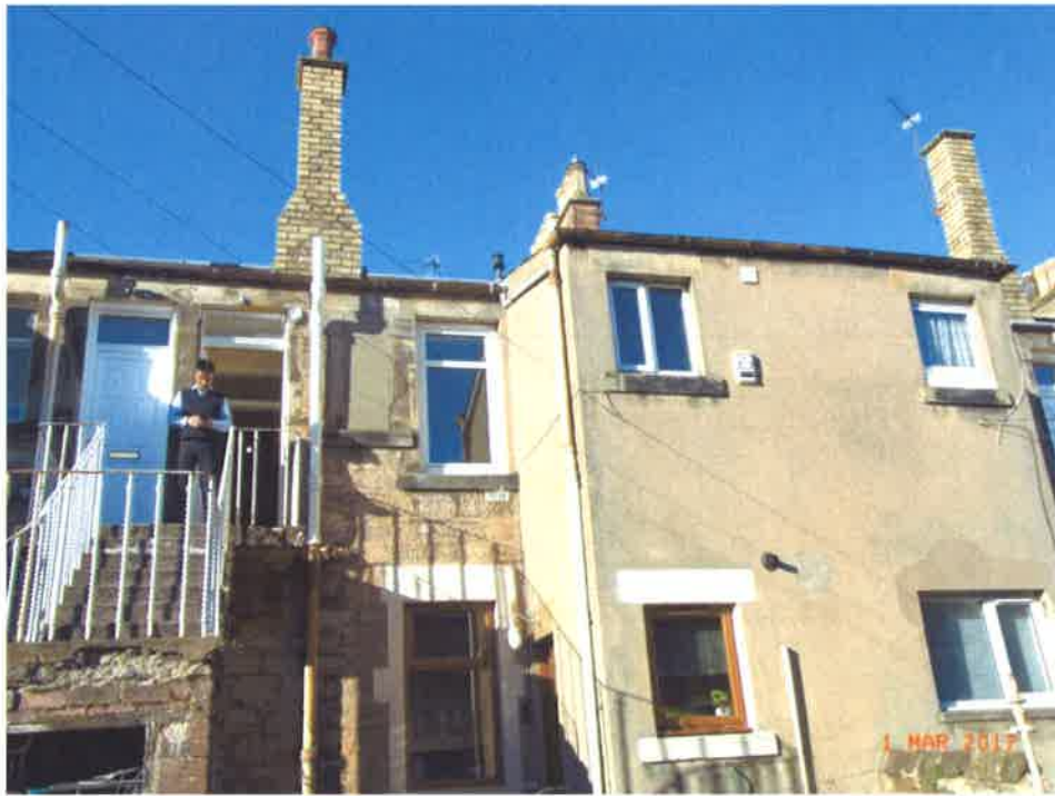
Rear elevation – showing roof covering and rhones
