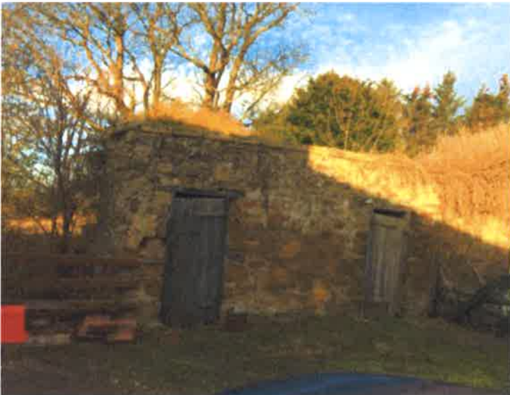
Stores (not part of tenancy) adjacent to cottages
