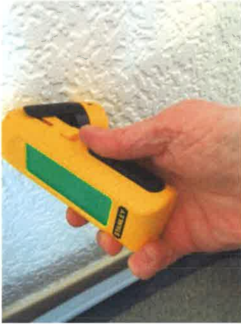
Damp meter reading taken under window in living room
