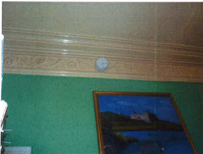
4. Hard wired smoke detector – living room
