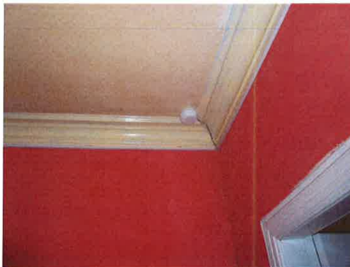
2. Hard wired smoke detector - hall
