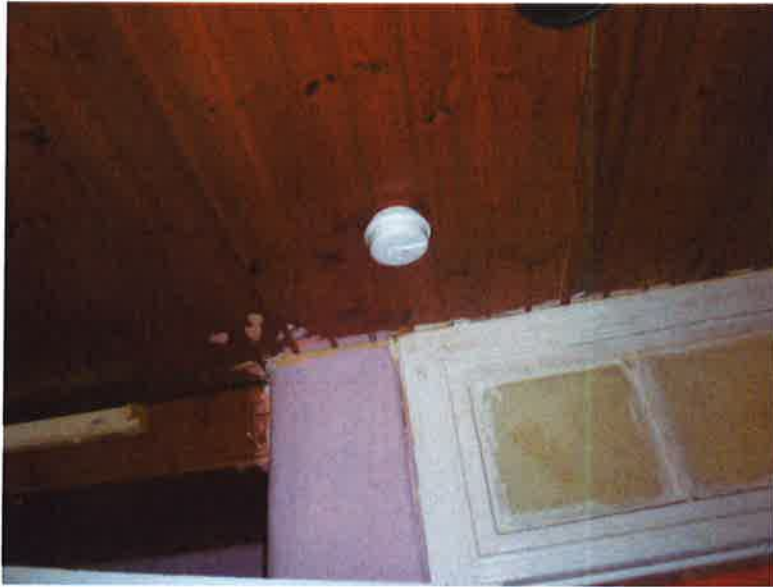
3. Hard wired heat detector - kitchen
