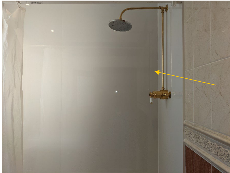
1 The new shower walls
