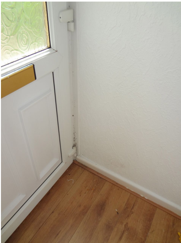
Walls/floor at front door
