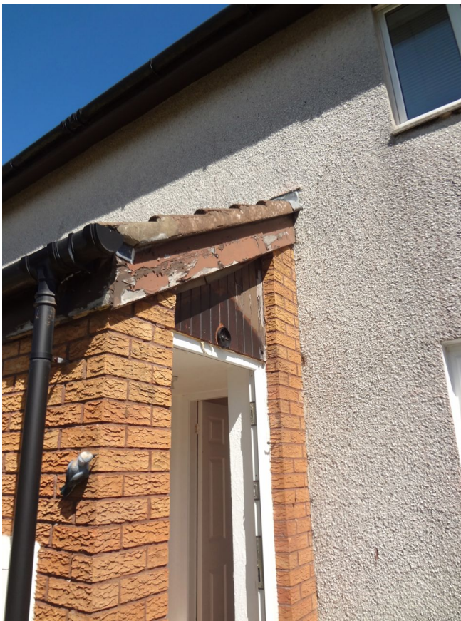
Damaged canopy at Front Door has been removed
