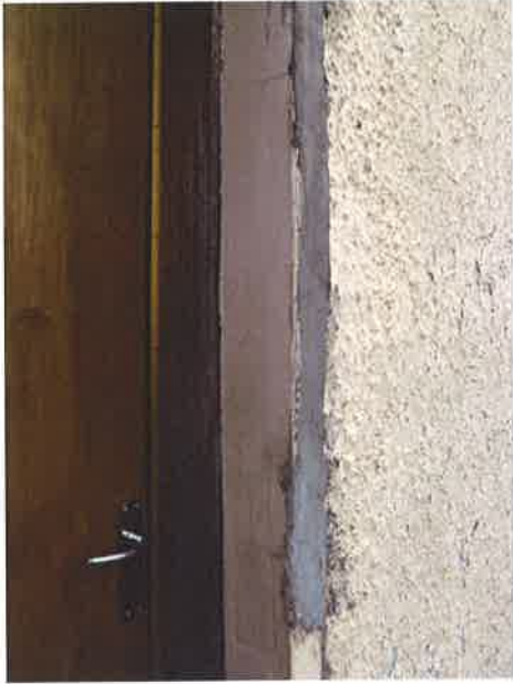
Render Repair 1 st February 2017
