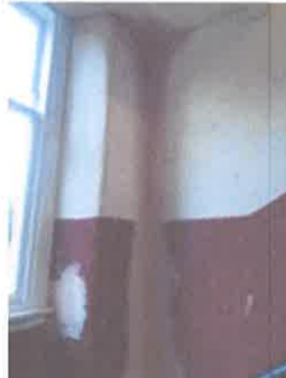
Exposed new plasterwork to communal close on half landing between ground floor and first floor
