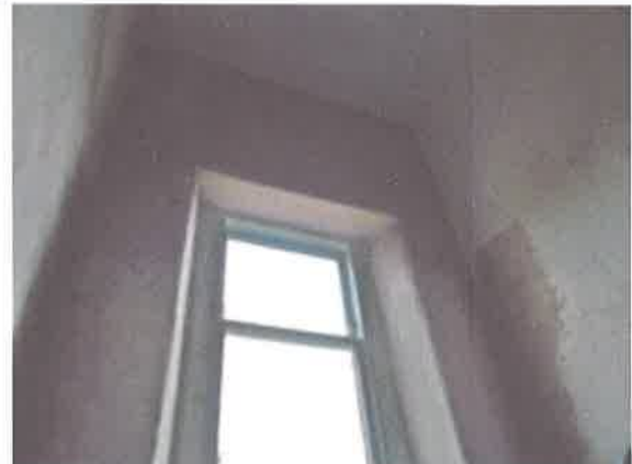
Exposed new plasterwork to communal close on half landing between first and second floor
