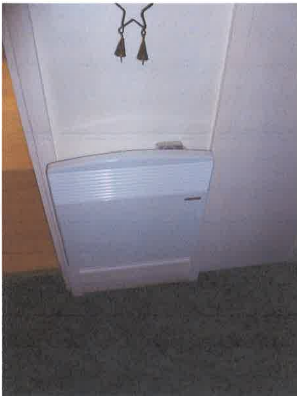
Electric panel heater hall - August 2017
