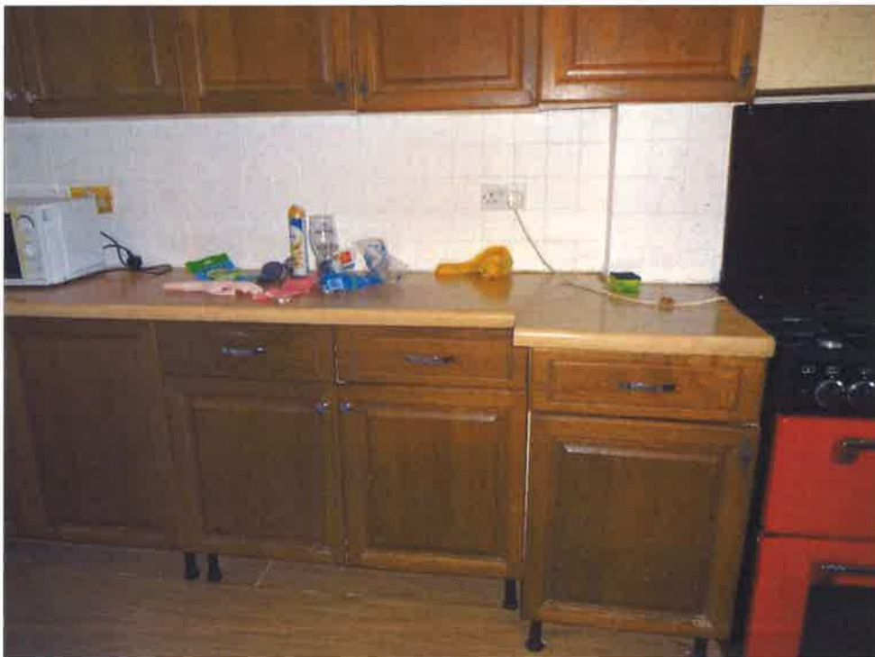
Kitchen drawers repaired
