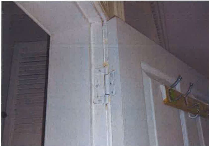
Replacement hinges fitted to bathroom door
