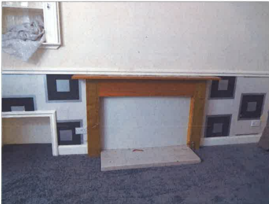
Gas fire removed from lounge and wall repaired
