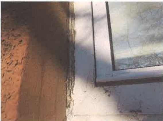
23 Cracked/split perimeter sealants.
