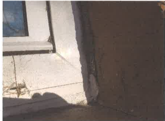
22 Close view of perimeter sealant to windows.
