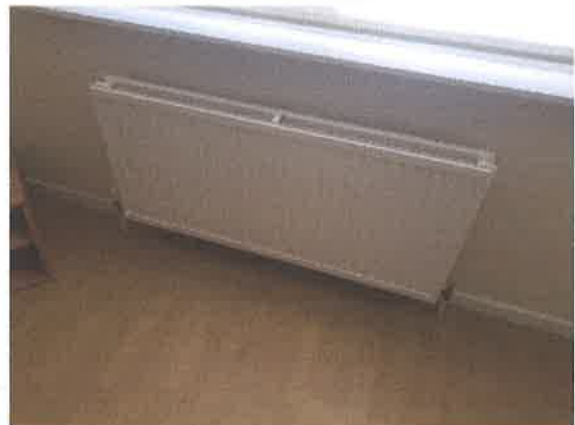
10 Metal pressed panel radiator - central heating.
