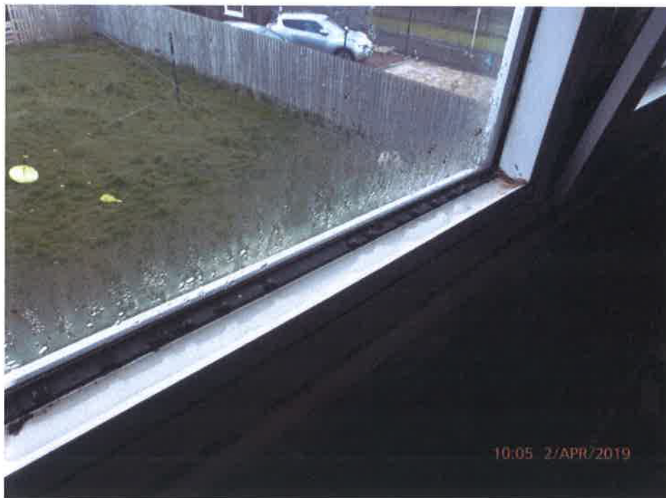
Condensation on the window
