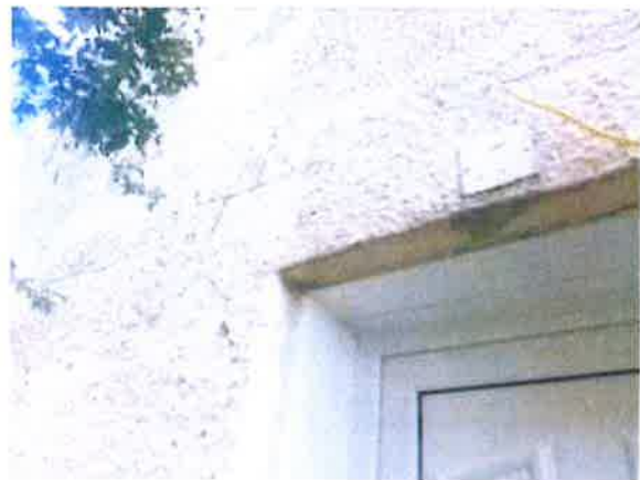
2 Gable Elevation – view of cracked render.
