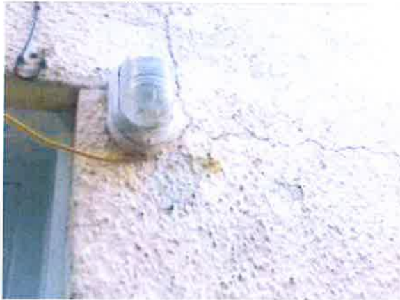
3 Gable elevation – view of cracked render.
