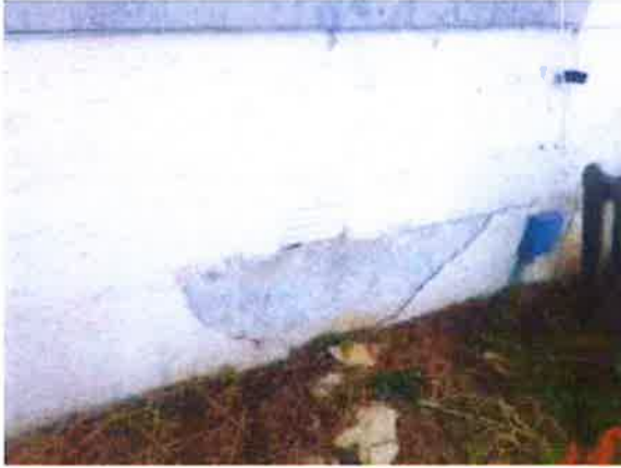
7 Defective render at Front Elevation.
