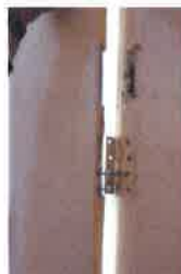
2c) Spare bedroom door as at 22/06/17 – door detached from hinges
