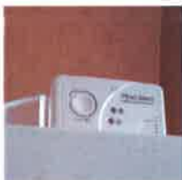
4a) As at 22/06/17 – Standing loose on fridge so does not meet regulations
