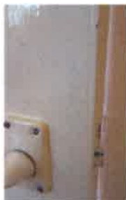
2a) Sitting room door as at 22/06/17 – door does not fit frame
