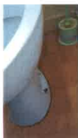
8a) As at 22/10/17 – not secured to floor
