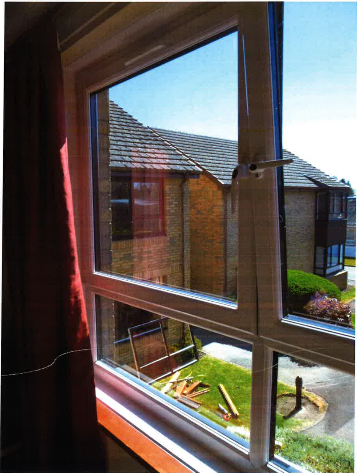
Lounge window internal – May 2017 New window
