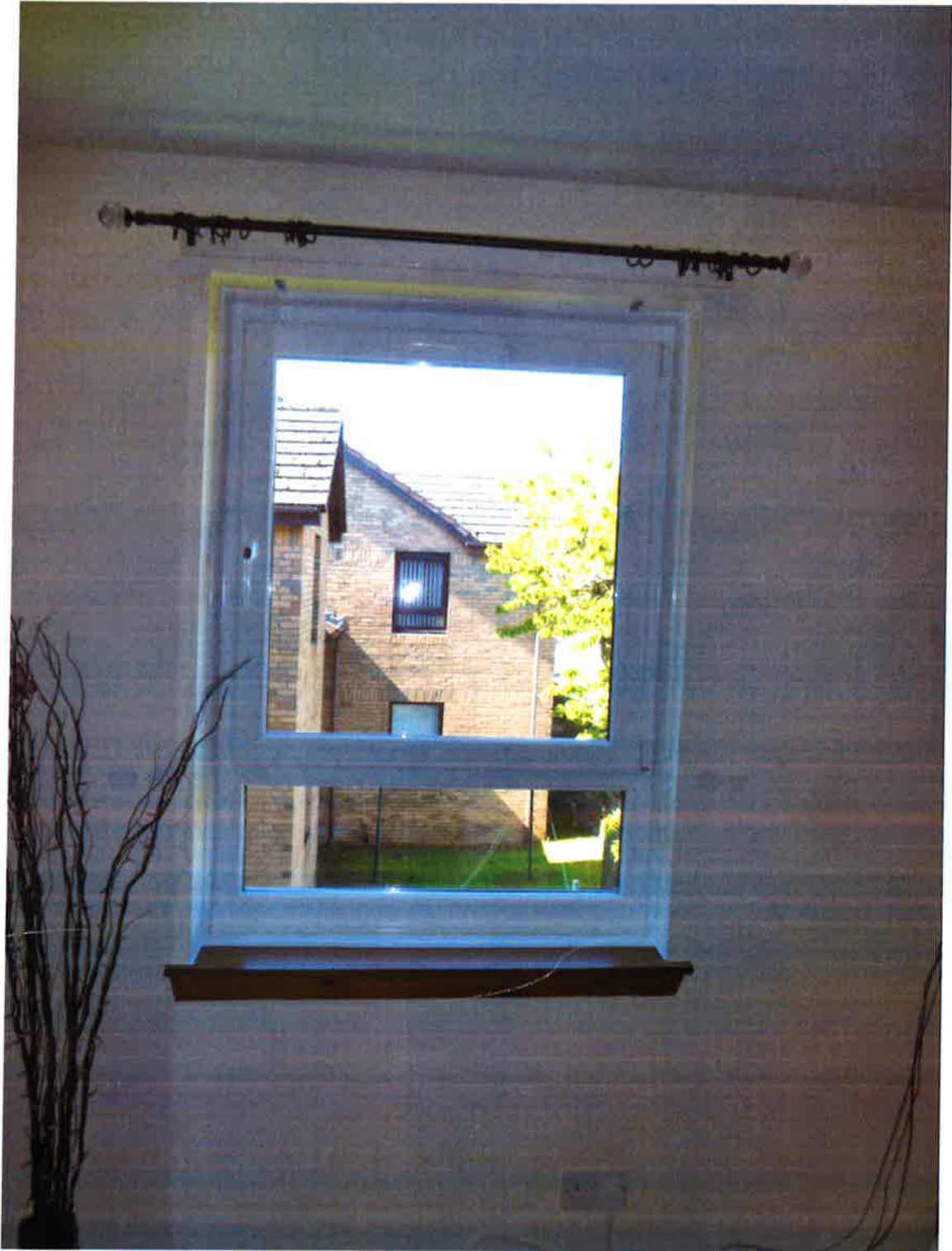
Kitchen Internal – May 2017 new window
