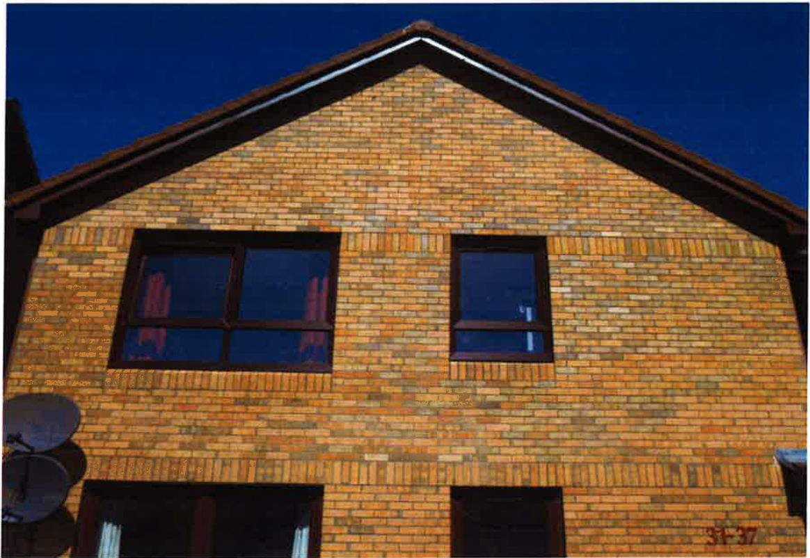
Lounge & Kitchen external – May 2017 new windows
