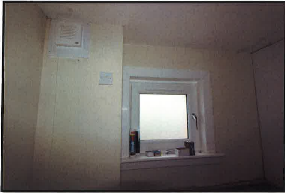
Photograph 6 Bathroom - new extractor fan and window.
