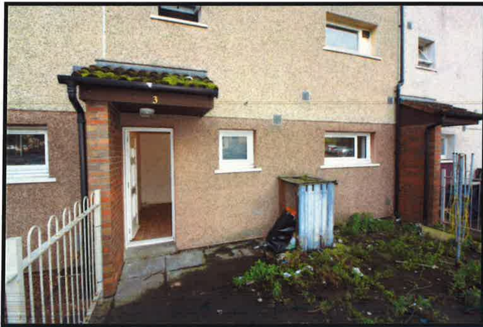
Photograph 1 Front Elevation - Front windows and door replaced.
