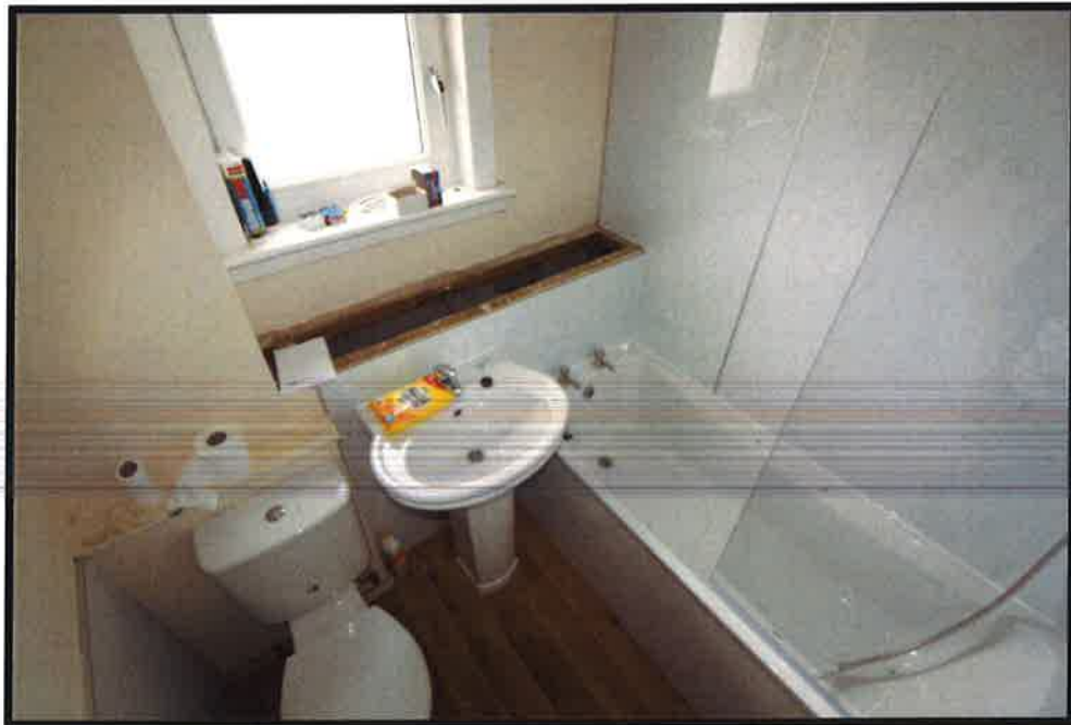
Photograph 5 Bathroom - new fittings.
