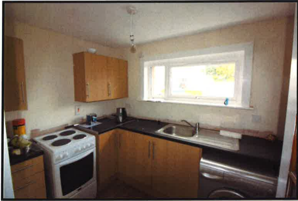
Photograph 4 Kitchen - New fittings. Extractor fan removed.
