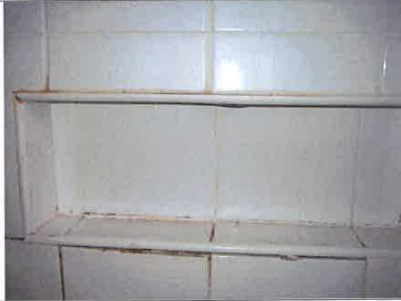
Poor grout to tiling
