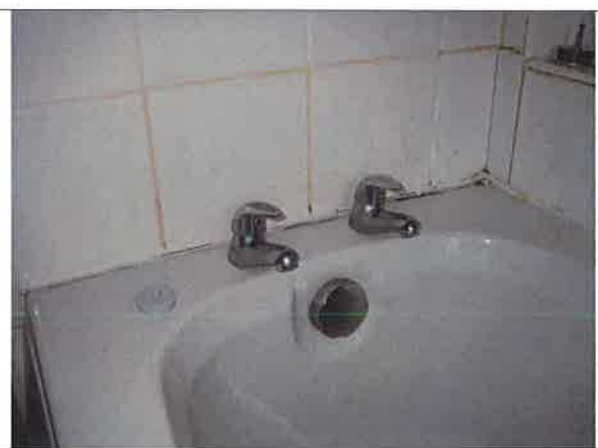
Bathroom seal poor
