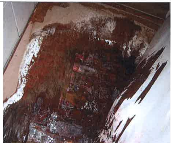
Bathroom floor wet rot
