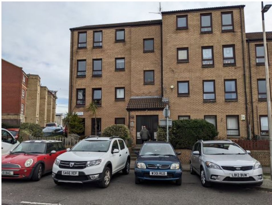
1 Front elevation 74/9 Restalrig Road South
