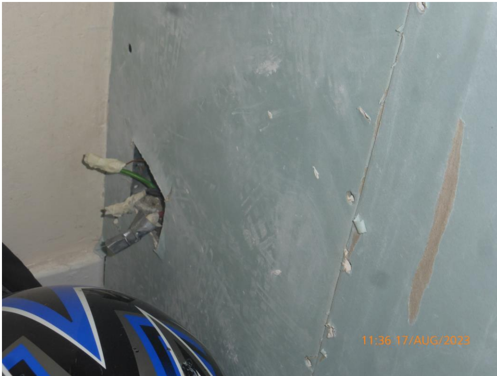
Exposed electrical wiring in the bedroom
