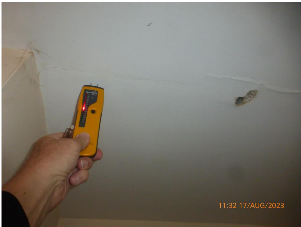
Damp stain and hole in the ceiling
