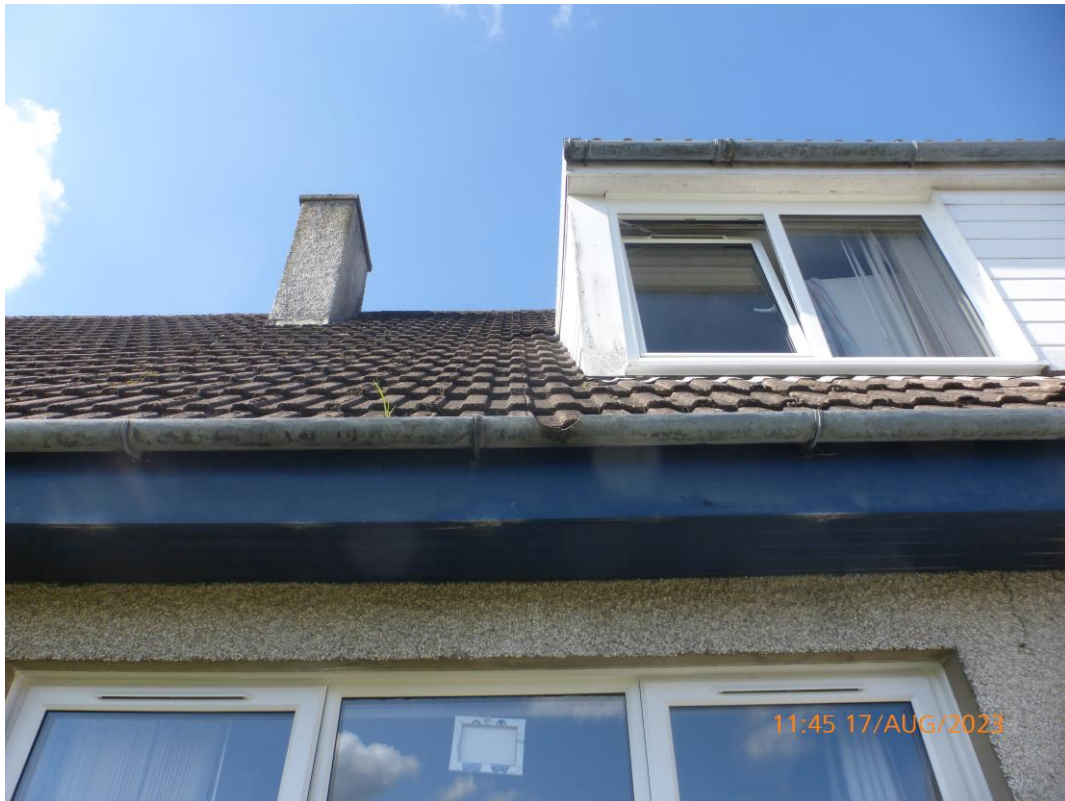
Broken front guttering
