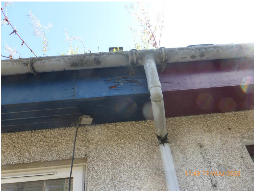
Rotten woodwork below choked rainwater fitting
