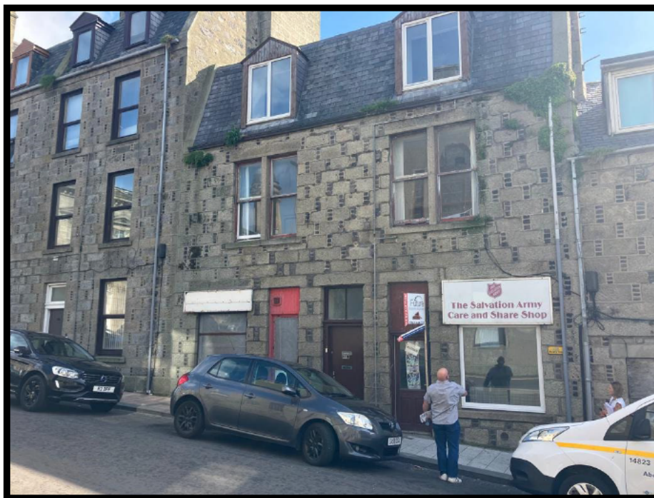
Photograph 1 Front (Western elevation): Communal entrance, first floor lounge and Bathroom windows, vegetation in rainwater goods.
