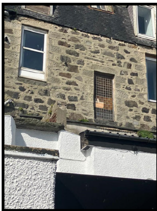
Photograph 4 Rear elevation: Damage to stairwell window, missing slates adjacent to top floor dormer.
