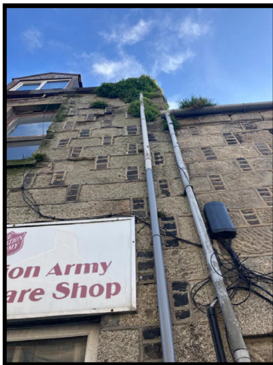
Photograph 3 Front elevation: Vegetation to rainwater goods and masonry.
