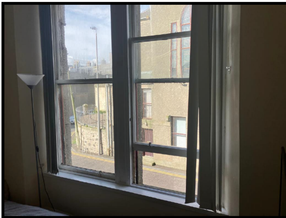
Photograph 8 Bedroom window: Overview, no method of restricting opening, low sill height
