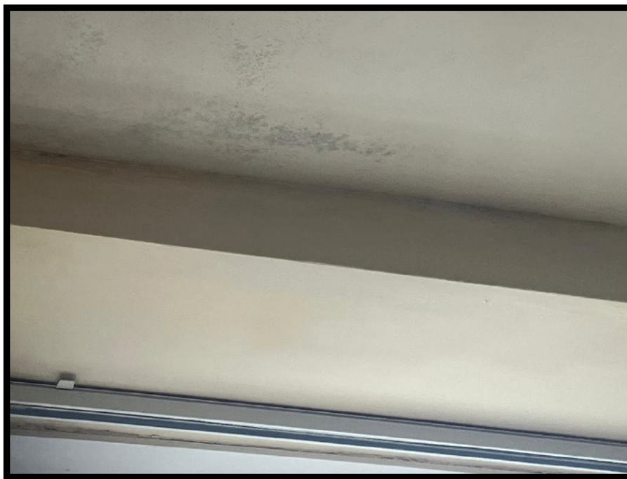
Photograph 12 Kitchen: Staining above window from previous damp ingress.
