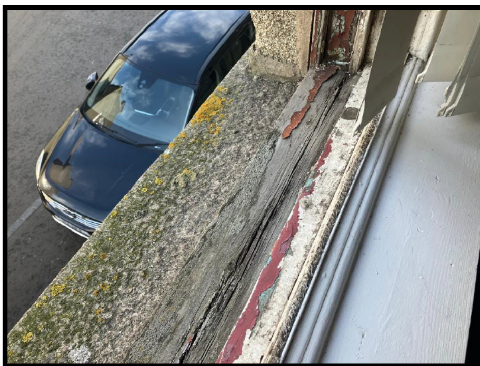
Photograph 9 Bedroom window: Rot to sill, weathered décor.
