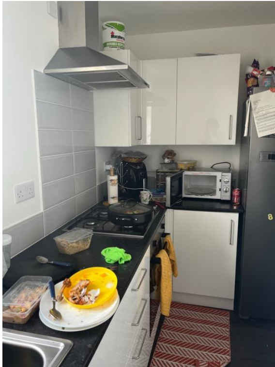
Photograph 6: Kitchen: replacement fittings including units and switches
