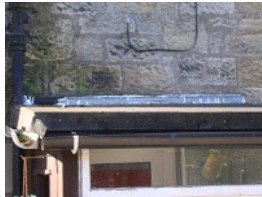
PORCH ROOF FLASHING/GUTTERS
