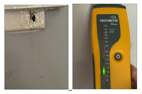
A hole has been drilled to accommodate a cable which is no longer in use. No evidence of water ingress was noted around the area of the drill site.
