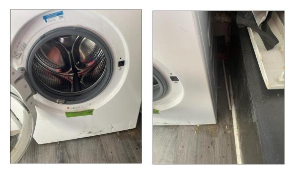
Washing machine was not tested during visit, however an area of water staining was noted at the righthand corner of the washing machine.
