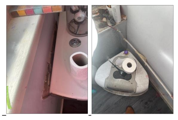
The toilet cistern has come away from the wall and the overflow pipe has been sealed with masking tape no leaks were noted.
