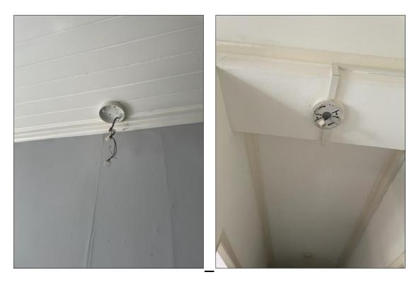
No working heat detector in kitchen. No working smoke detector in hall
