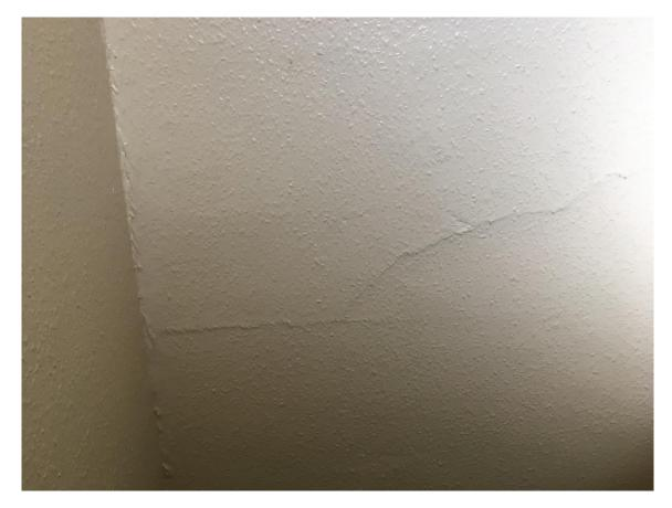
Horizontal cracking to plasterwork in stairwell.
