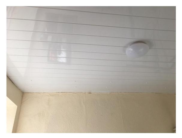
Recently reclad Bathroom ceiling. Moderate damp meter readings obtained on west wall.
