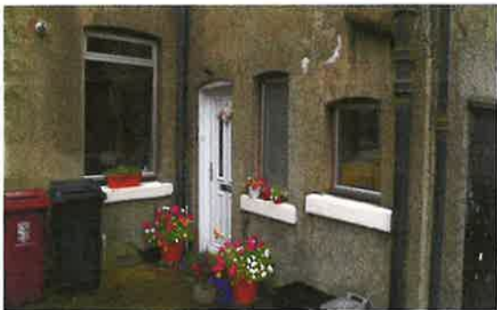
Photo 2 – Main door access on rear elevation
