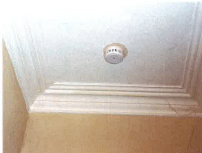
Photograph 8:- Landing smoke detector
