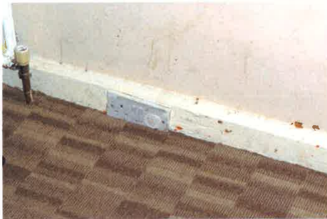
Photographs 7 & 8:- Low mounted power points
