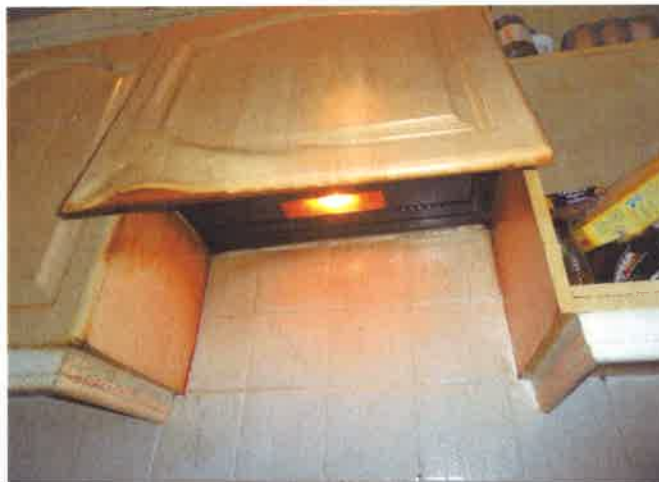
Photograph 5:- Warped kitchen fittings
