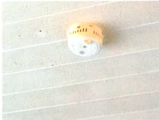
Photograph 7 :- Heat detector - kitchen
