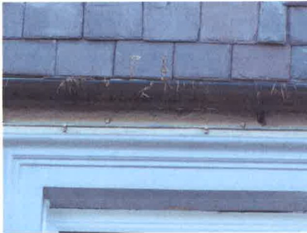
Photograph 3:- Dead Vegetation in PVC guttering
