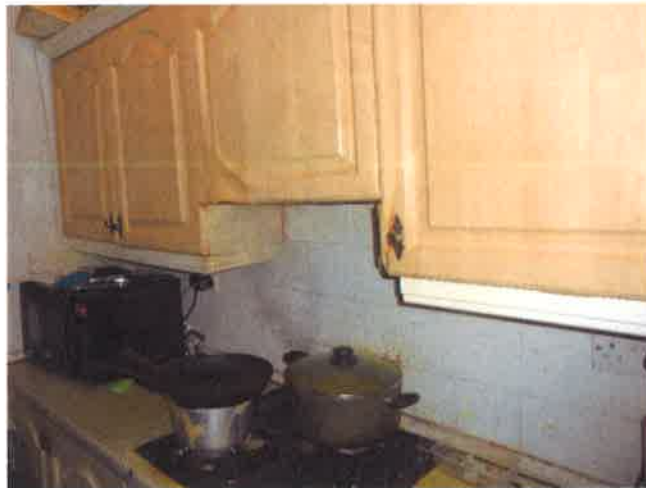
Photograph 4:- Warped kitchen fittings
