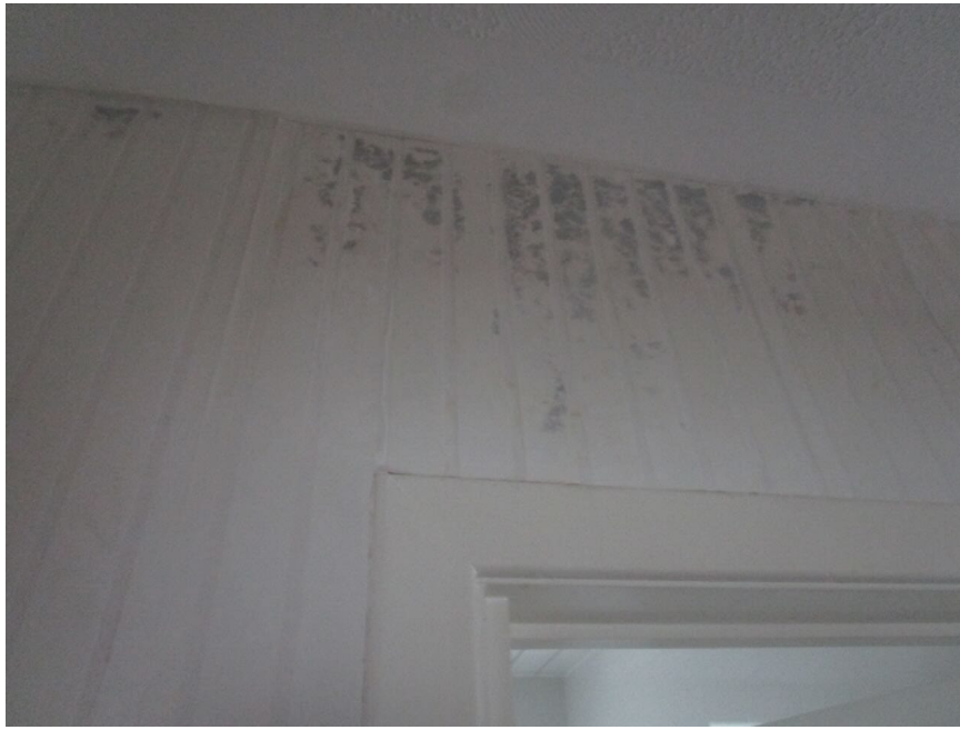
1. Water damage on hall wall/ceiling adjacent bathroom door
