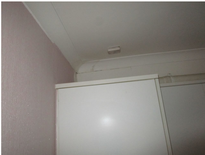
4. Historic water damage in kitchen at cornice
