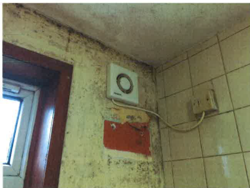
1 The mould growth in the bathroom at the rear wall and the inoperative extract fan
