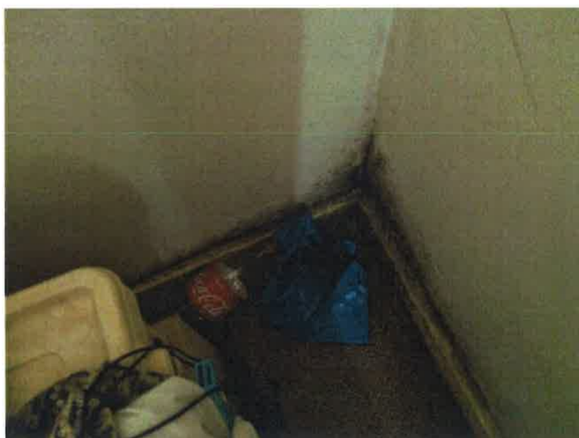
3 The mould growth in the corner of the rear bedroom
