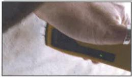
Water damage was noted to the common stairwell which appears to have been due to water leaking from a damaged pipe within the main bathroom of flat 3/1.
