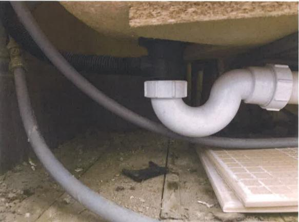
Shower was recently replaced and tiles made good. No evidence of water ingress or dampness behind the bath panel.
