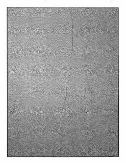
Areas of cracking are visible on the walls and ceiling this appears to be superficial.
