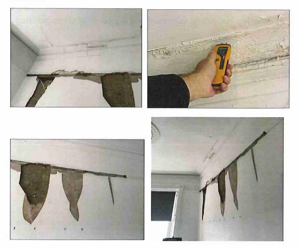
Large sections of plaster have been removed by contractors along the lounge wall and cracks are visible at the kitchen area.
