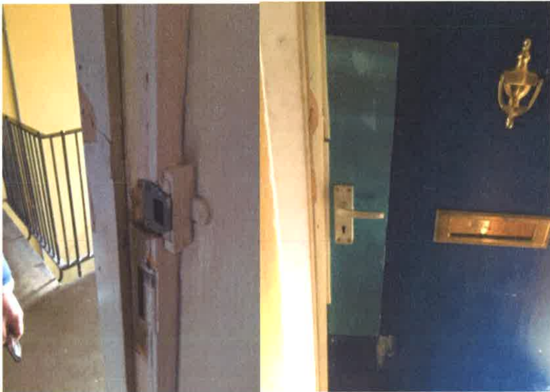
Front Door - showing new mortice lock and door secured
