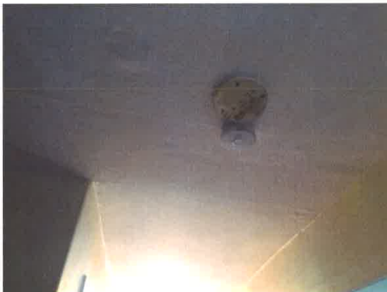
Smoke detectors – battery detectors fitted in kitchen and hall
