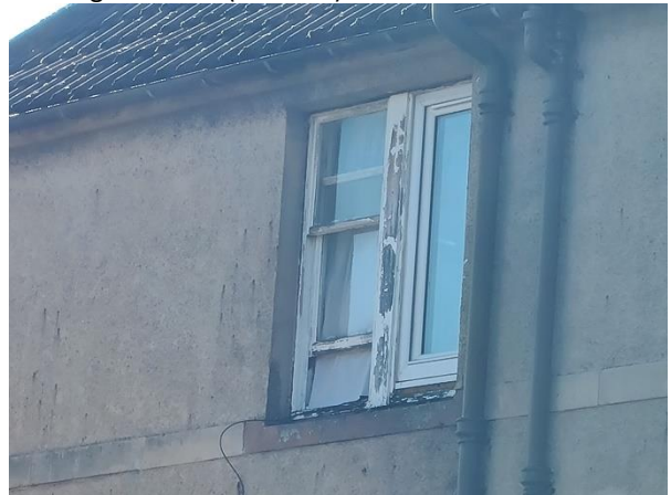
4 Bathroom window (external)
