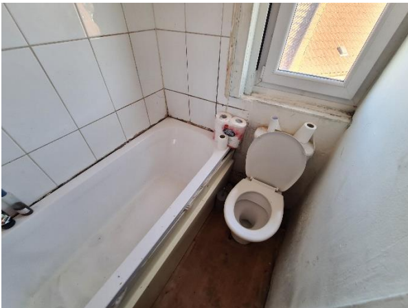
17 General view of Bathroom.
