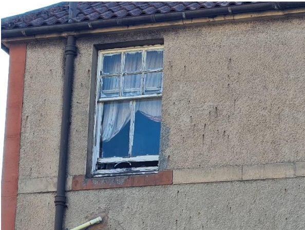
3 Kitchen window (external).
