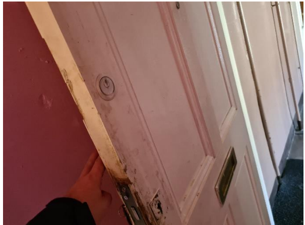
28 Entrance door – external face.
