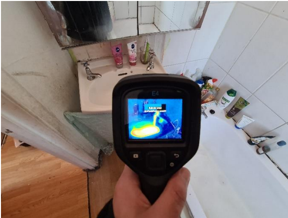
13 Hot water to wash basin.
