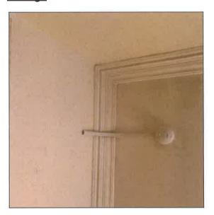
Smoke detector fitted and tested - linked with hall smoke detector but not linked with heat detector in kitchen.
