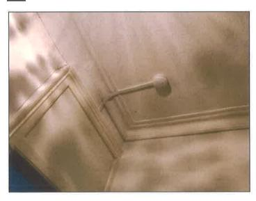
Smoke detector fitted and tested - linked with lounge smoke detector but not linked with kitchen heat detector.
