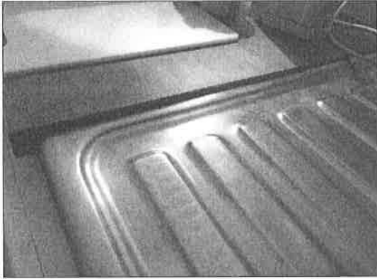
Sink and drainer unit is not attached to base and is not supported
