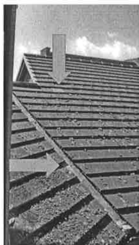
1a) As at 17/08/17 – detail of valley gutter and replacement tiles.
