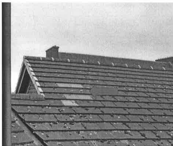
12) As at 20/09/17 – detail of further replacement tiles
