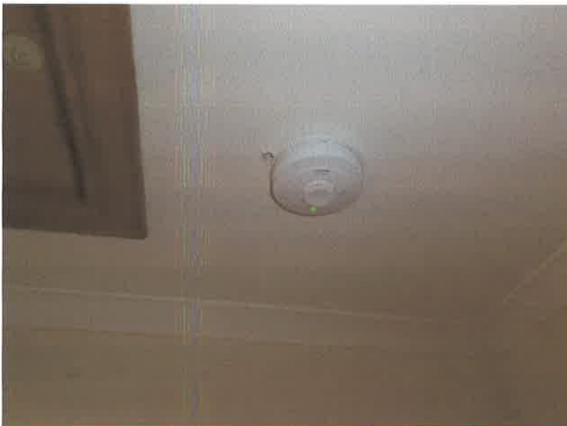
Combined smoke and CO alarm on landing
