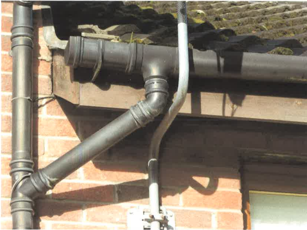
Rhone and downpipe properly connected
