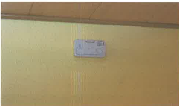
Carbon Monoxide alarm in kitchen above gas boiler
