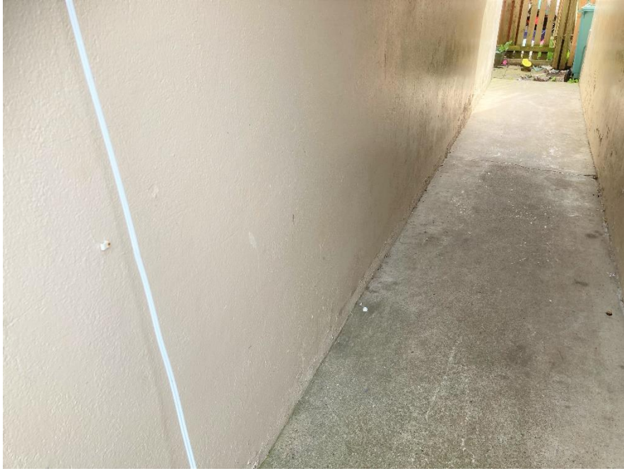
28 Flaking paint and general staining pend wall – no significant defects evident
