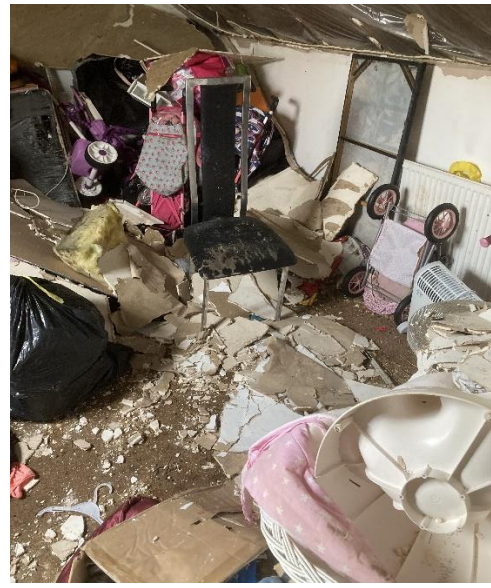
7. Floored and lined attic
