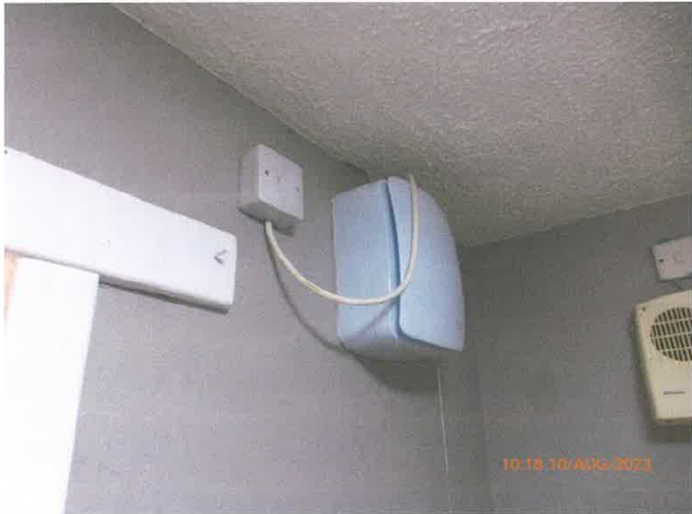
New extractor fan in the Bathroom
