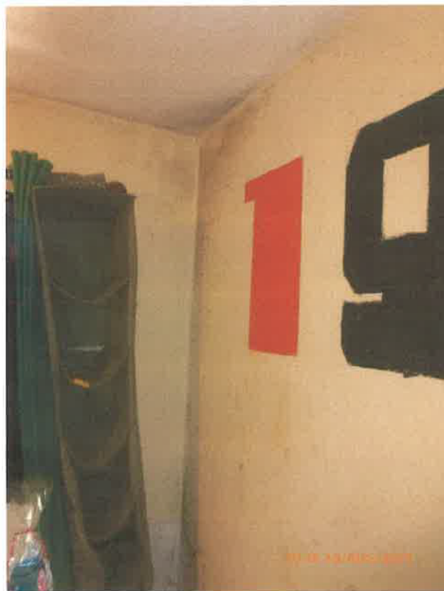
Mould and staining in the small Bedroom
