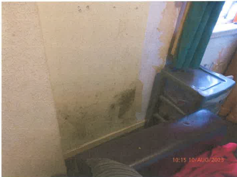
Mould and staining in the small Bedroom
