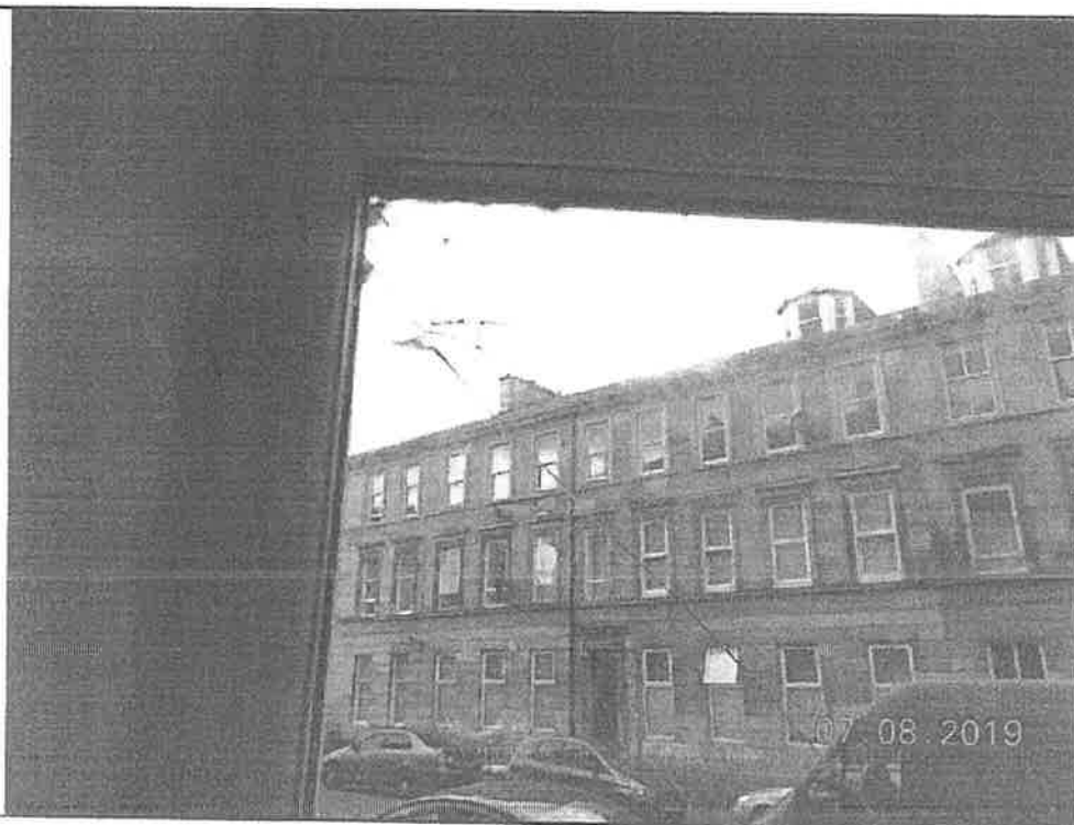
10. Cracked glass from inside
