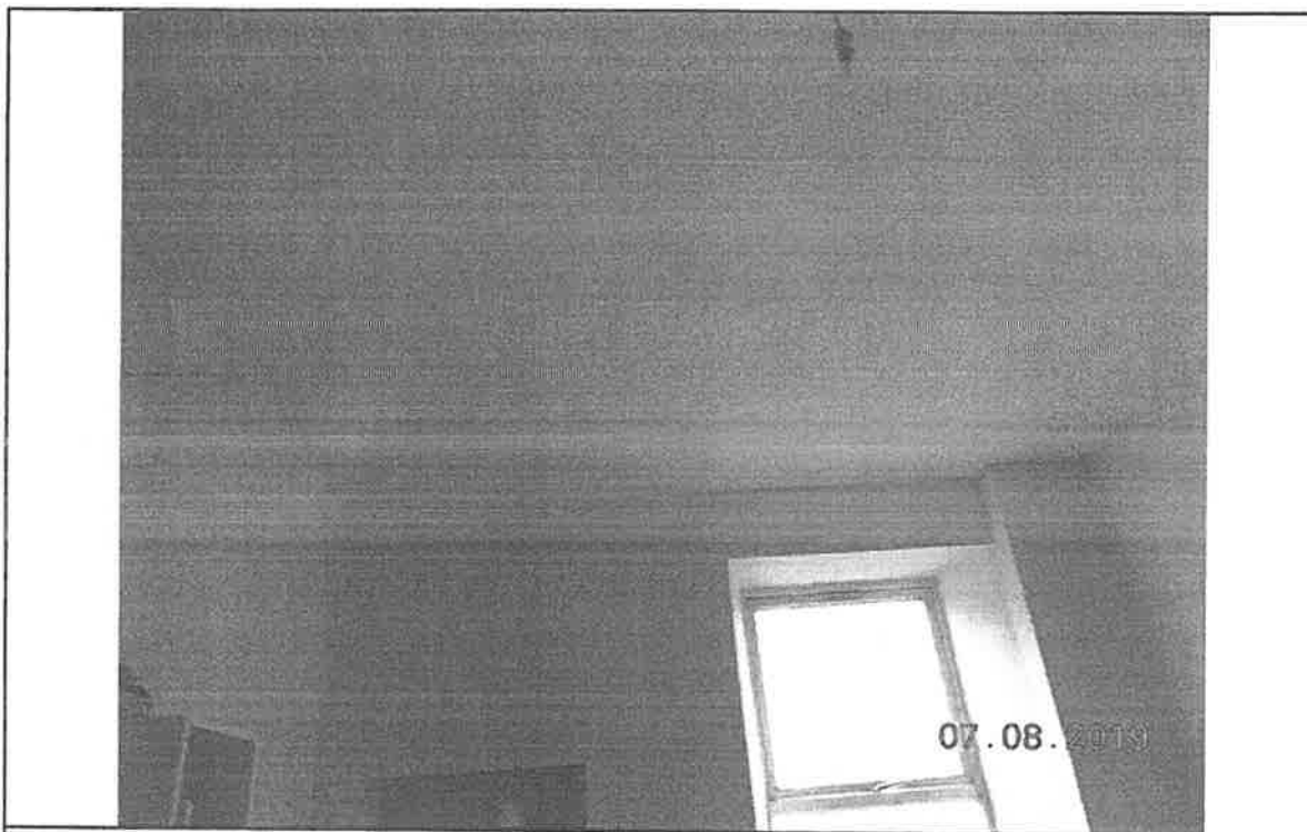
5. Ceiling in Kitchen
